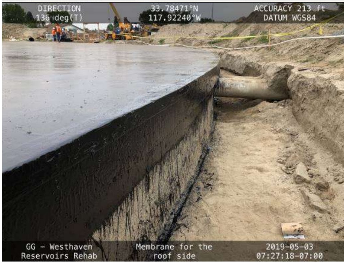
Membrane for the Roof Side
