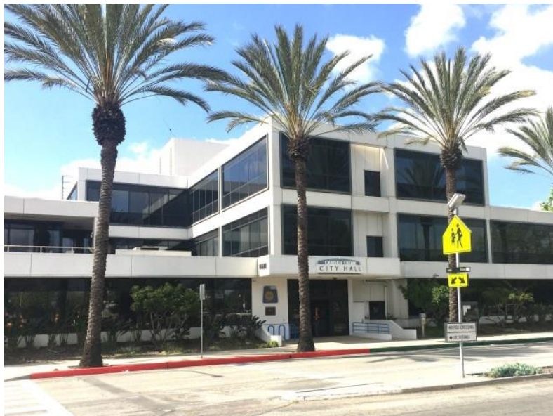
GARDEN GROVE City Hall (Orange County Tribune photo).
