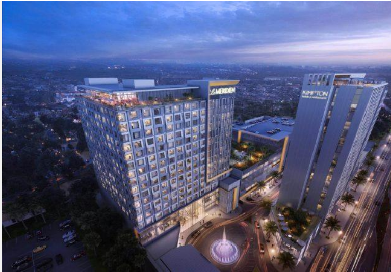
THE AURELA project, with Kimpton and LeMeridien hotels on Harbor Boulevard (City of Garden Grove).
