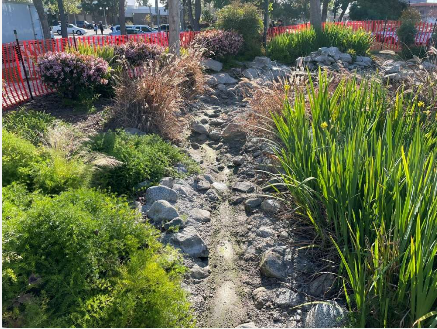
Photo 3. Dewatered section of the pond.
