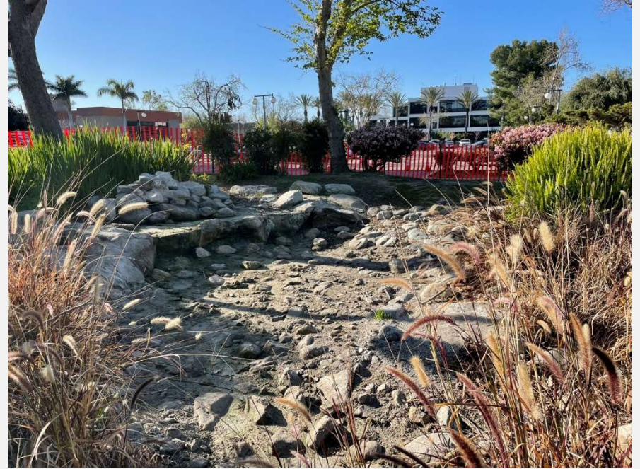
Photo 4. Dewatered section of the pond.
