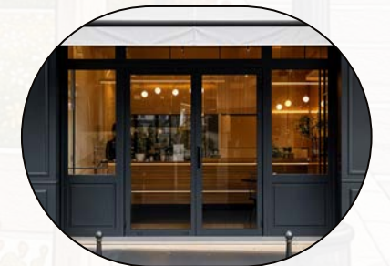
Traditional (Fixed Glazing & Display Window)
