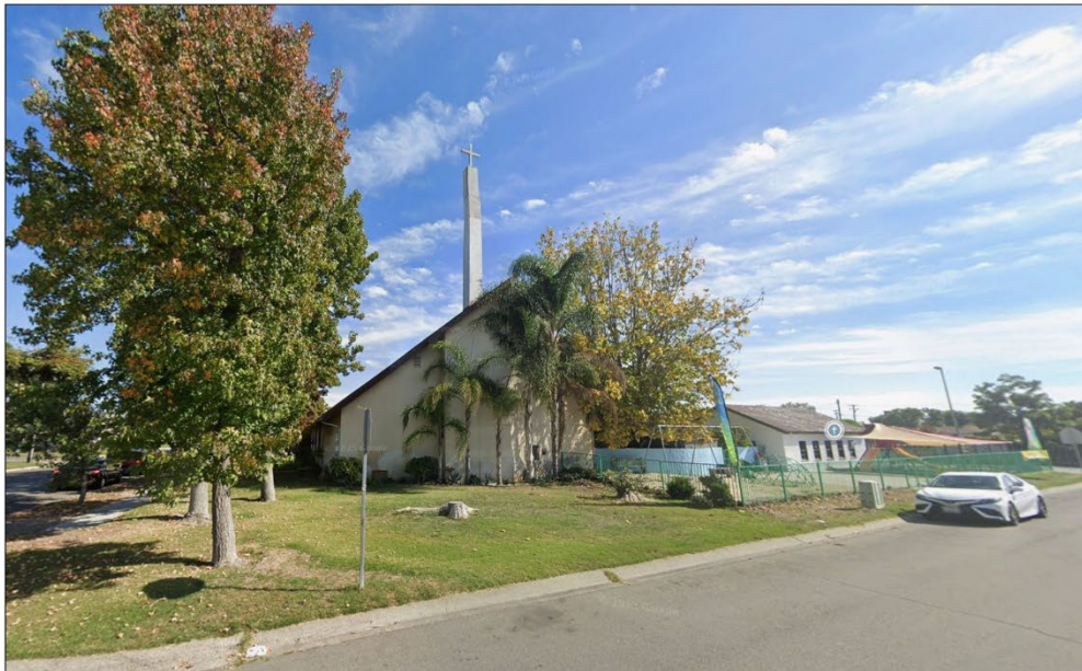
View of the Project Site from Kerry St Facing Southeast
