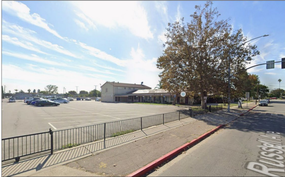
View of the Project Site from Russell Ave Facing Southwest
