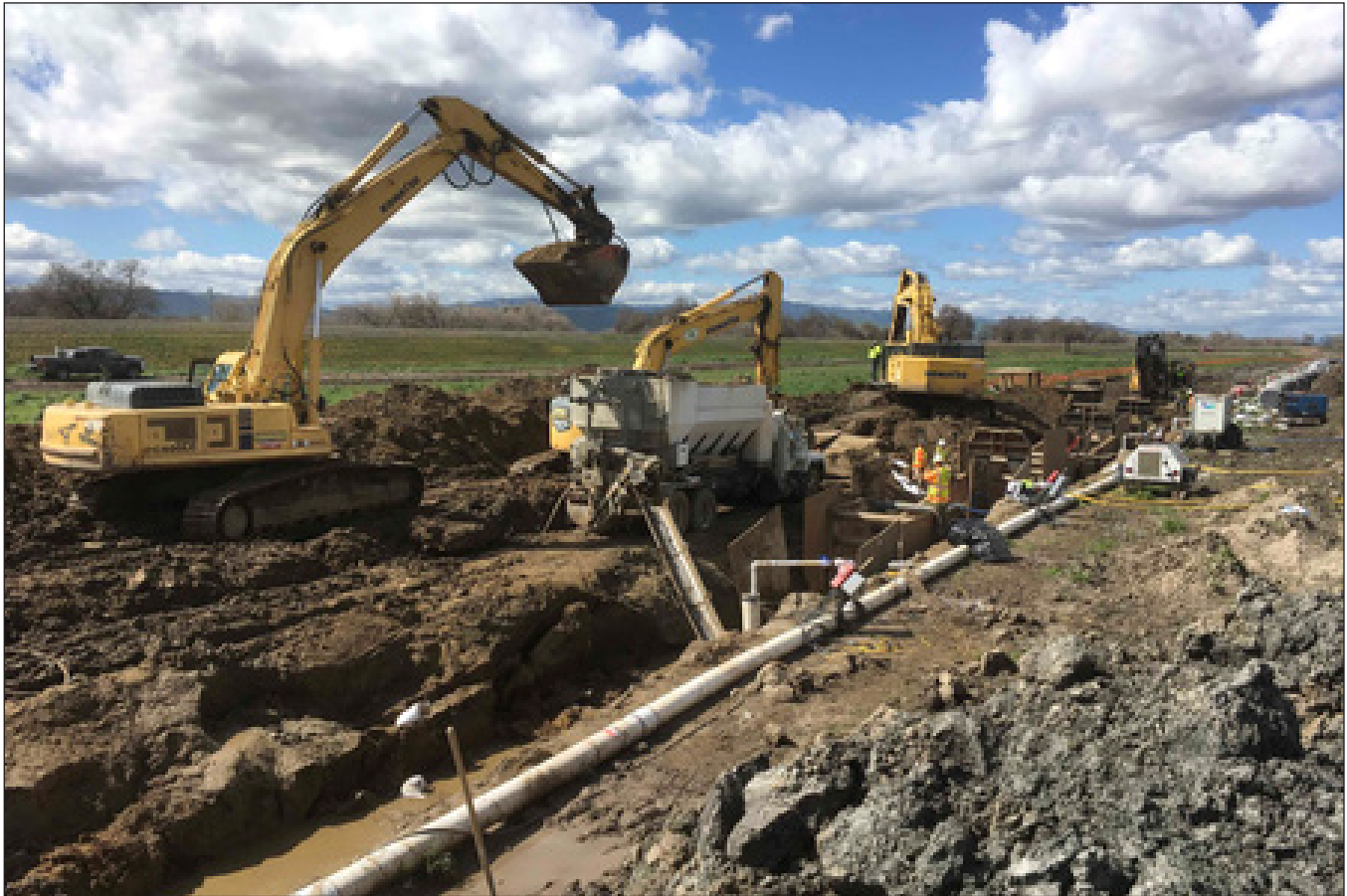
This $28 million recycled water pipeline project was constructed to convey Title 22 recycled wastewater from the City of Turlock's outfall location at the San Joaquin River to the City of Modesto's effluent pump station location about 7 miles away.
