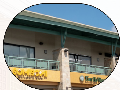
Continuous Building Overhang
