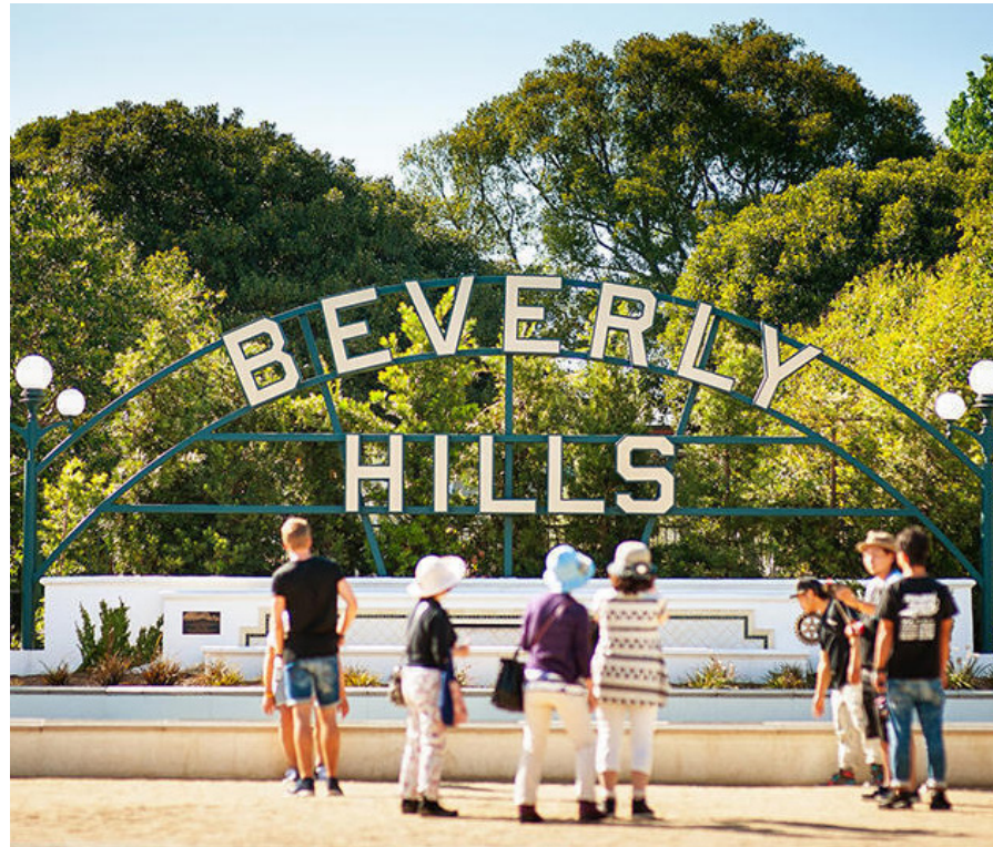
Arched monument sign featuring large district lettering on a structural steel frame.
