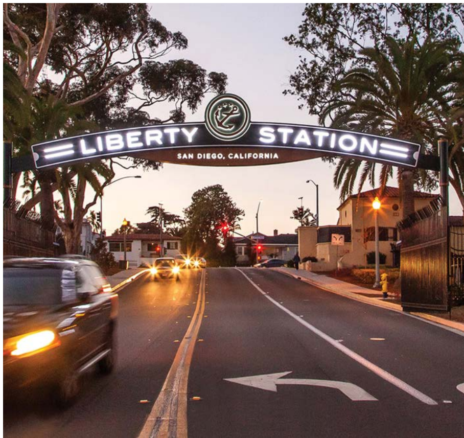
Gateway with illuminated channel lettering, integrated LED lighting, and a prominent district emblem.
