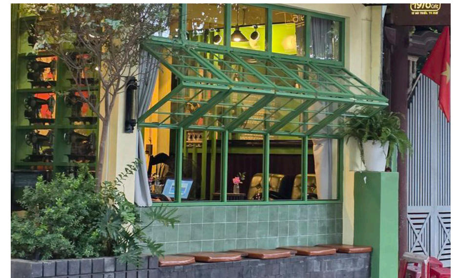
Operable awning windows integrated into a transparent storefront.
