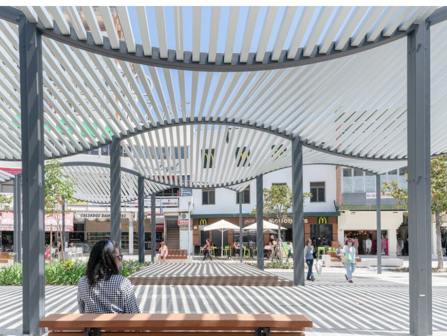
Louvered canopy providing filtered shade while maintaining natural light and ventilation in public spaces.
