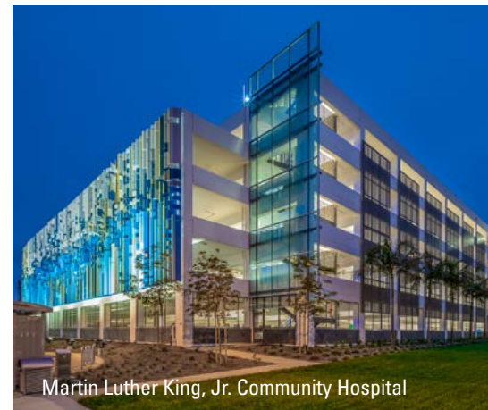
East County Parking Structure
