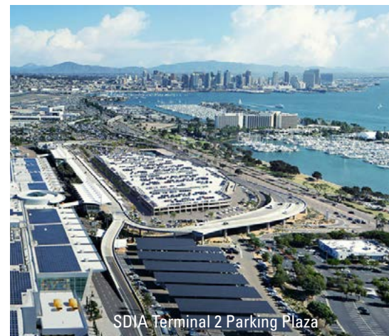
SDIA Terminal 2 Parking Plaza
