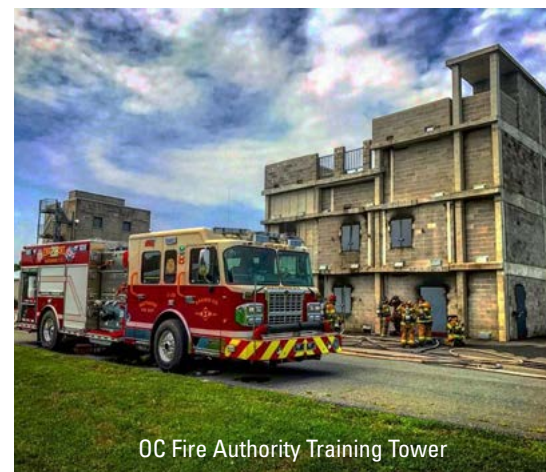
OC Fire Authority Training Tower
