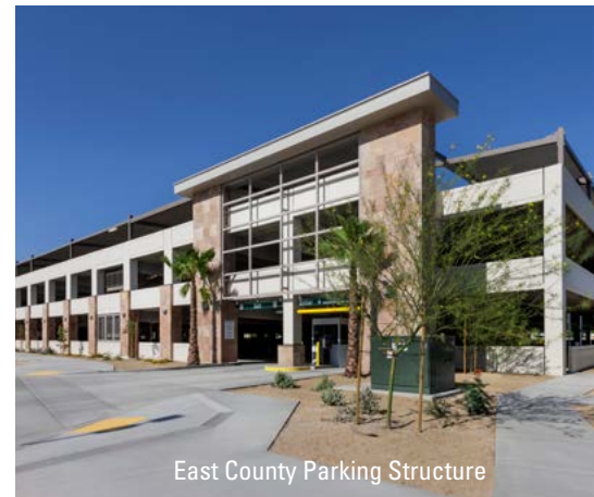
East County Parking Structure
