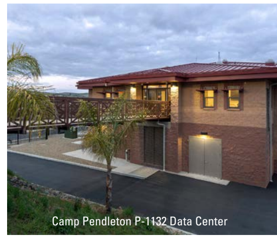
Camp Pendleton P-1132 Data Center
