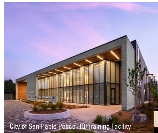
City of San Pablo Police HQ/Training Facility
