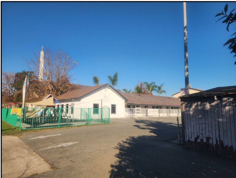
Plate 3.2-2: Overview of the 9822 Russell Avenue buildings from the southwest corner of the project, facing northeast.
