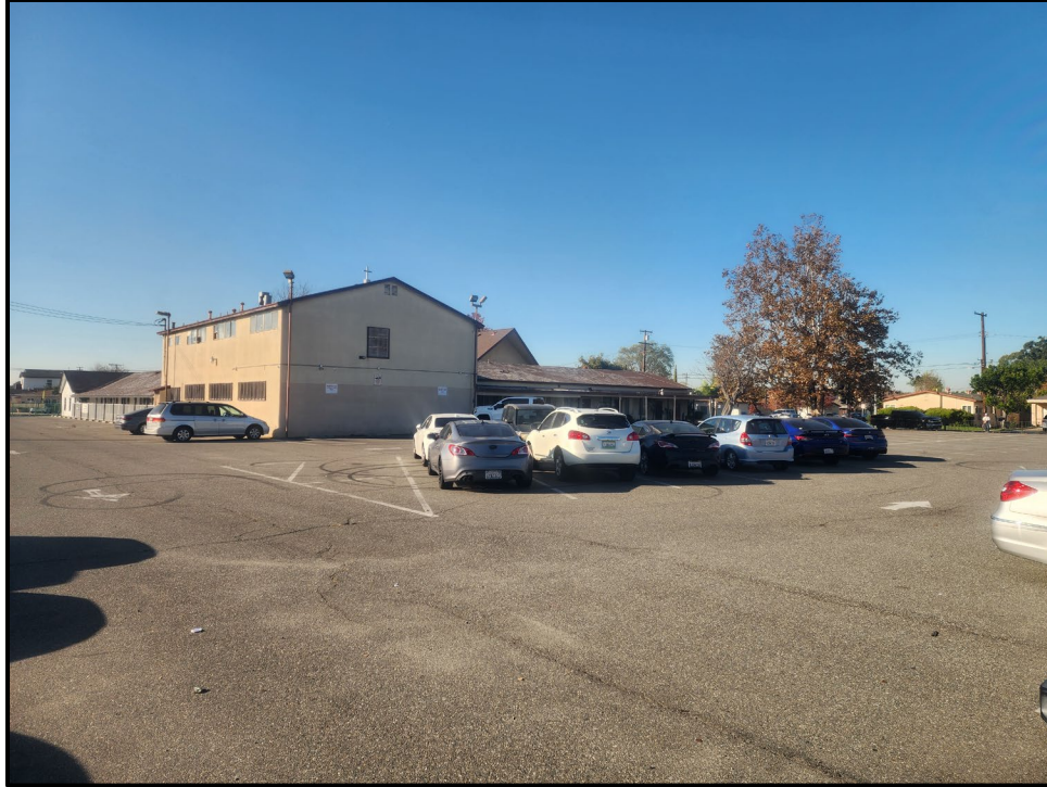
Plate 3.2-3: Overview of the 9822 Russell Avenue buildings from the southeast corner of the project, facing northwest.
