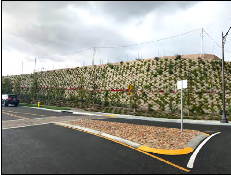
Northerly terrace retaining wall.
