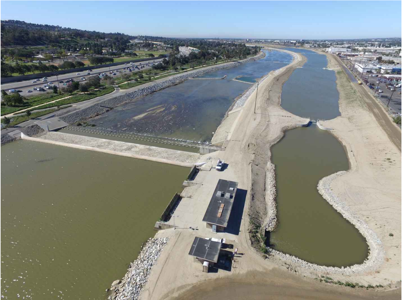
Figure 14-1: View of Santa Ana River (left) with OCWD recharge facilities (right). An inflatable rubber dam that crosses the river here enables OCWD to divert some river flows into basins for percolation.
