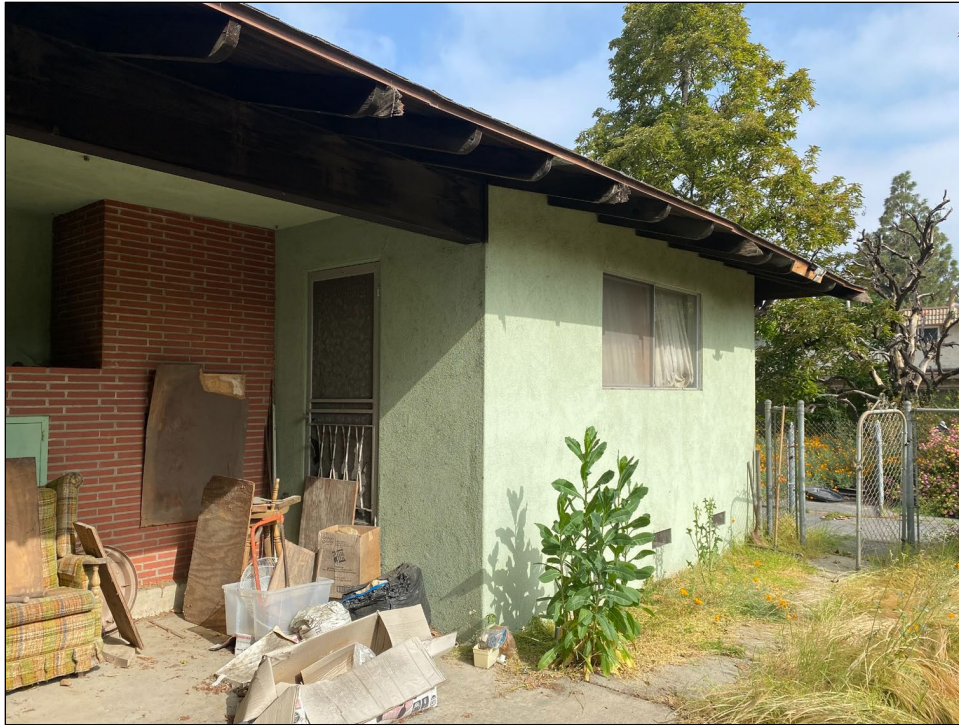
Figure 11. Exterior of Existing House
