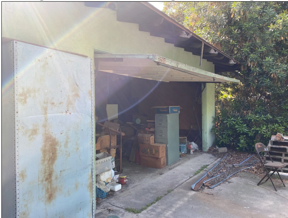
Figure 12. Exterior of Existing Attached Garage
