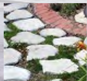
Permeable pavement allows water runoff to infiltrate through the soil and prevents most pollutants from reaching the storm drain system.
