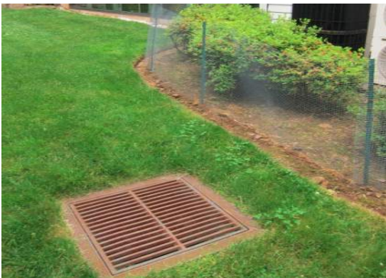
Fig. 2. Dry well installed to receive runoff flowing through a lawn (Source: R. Pitt)
