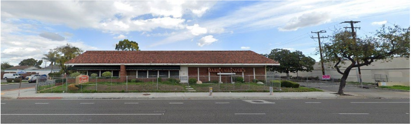
Views of the project site from Brookhurst Street.
