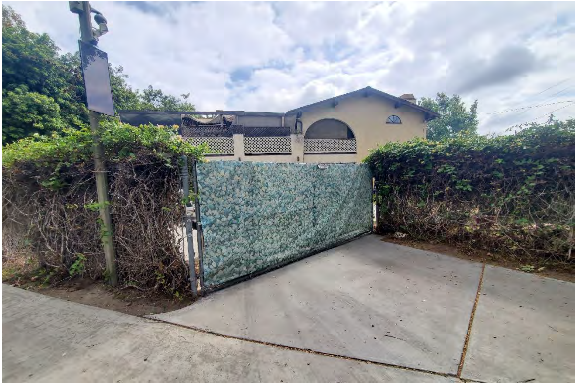
Photograph No. 3: Southeastern residential building, looking northeast (9091 Lampson Avenue).
