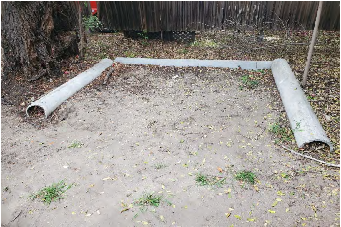
Photograph No. 9: Suspect asbestos-containing pipe (ACP) located in the yard (9081 Lampson Avenue).
