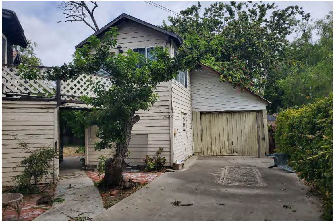
Photograph No. 7: Detached garage, with concrete patch noted in driveway (9081 Lampson Avenue).
