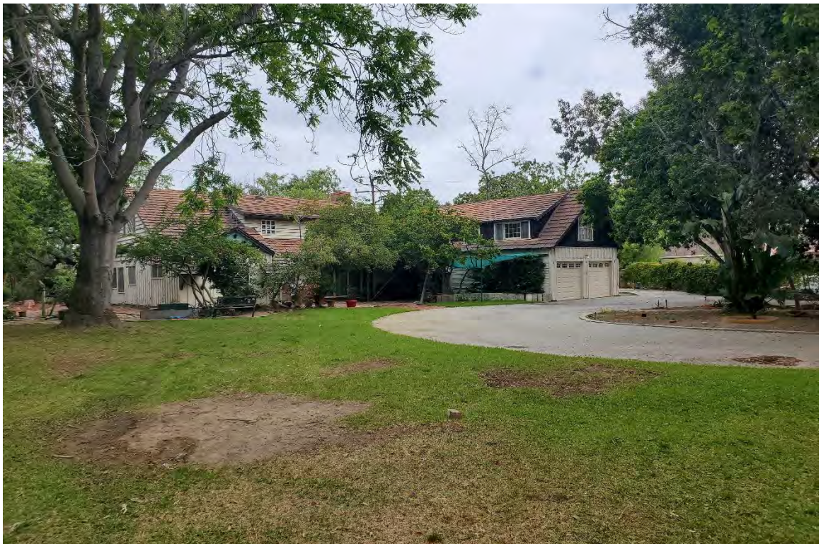
Photograph No. 6: Residential building, looking northeast (9081 Lampson Avenue).
