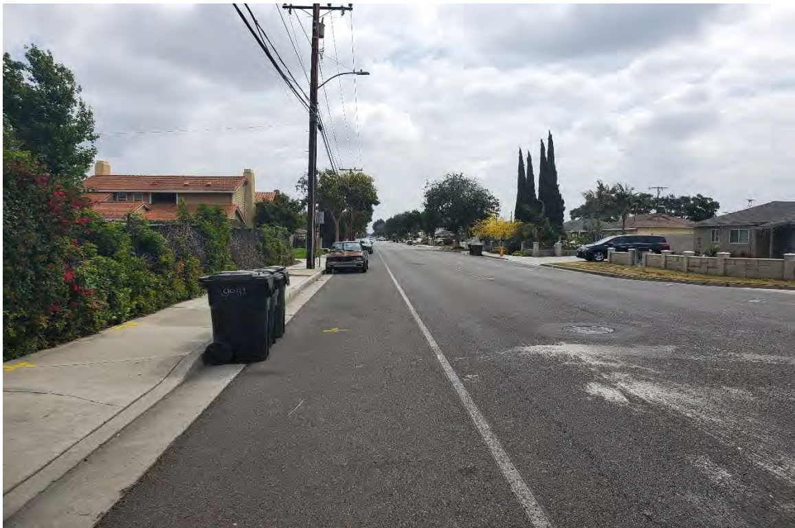
Photograph No. 12: Lampson Avenue, looking east, with view of pole-mounted electrical transformer located along site boundary.
