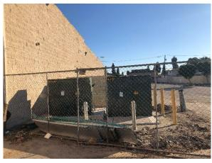
Photo #27 View of the two pad-mounted transformers located on the northwestern portion of the site.
