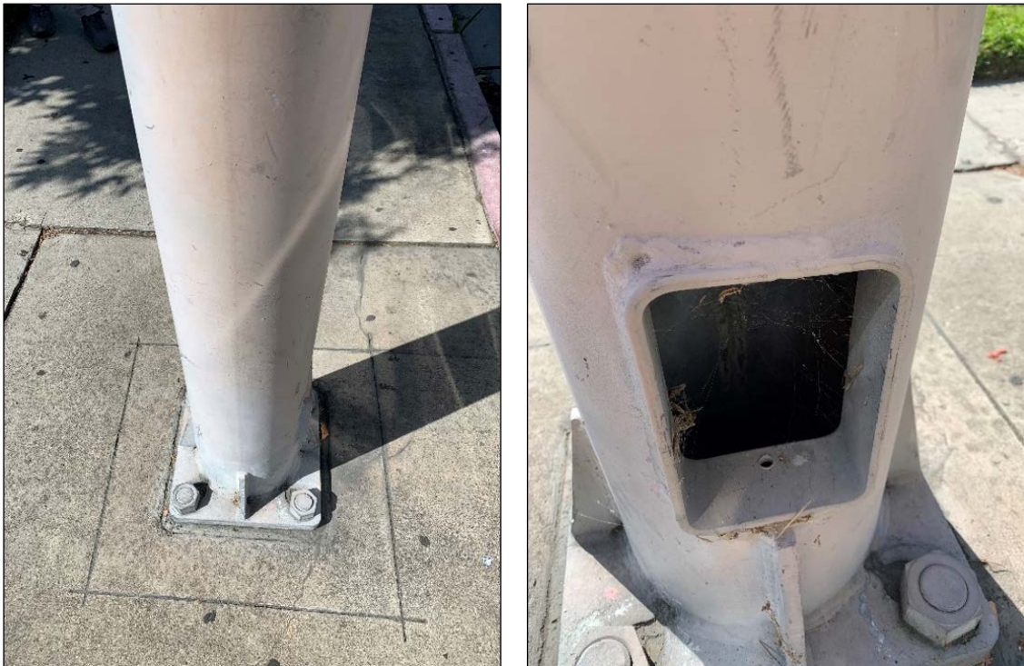
Figure 12 – South Banner Pole, Site #5
