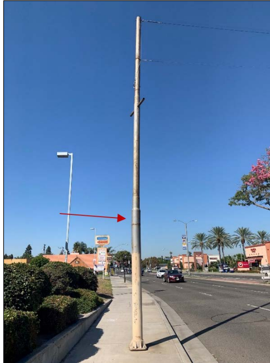
Figure 10 – Bend in South Banner Pole, Site #4
