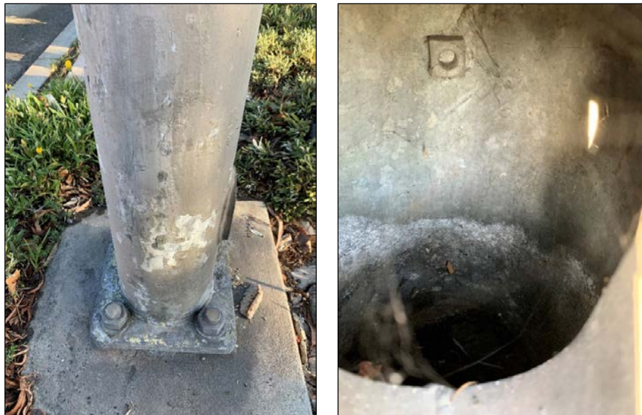
Figure 5 – Exterior and Interior Surfaces of Median Banner Pole, Site #2
