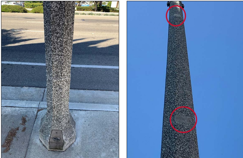
Figure 13 – Cast Concrete Banner Pole, Site #6
