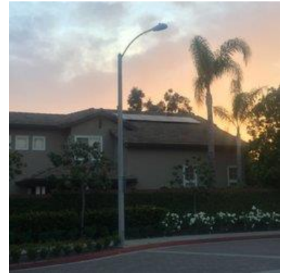
Tanko Lighting's Project in Orange, CA
