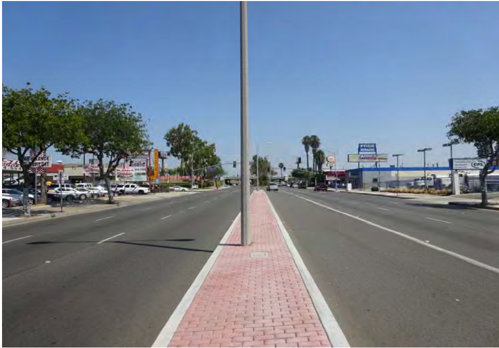
STREET SCENE 1: View looking north along Harbor Boulevard from the subject frontage.
