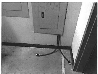
Maintain wiring in good condition and protect from damage. CFC 605.5
