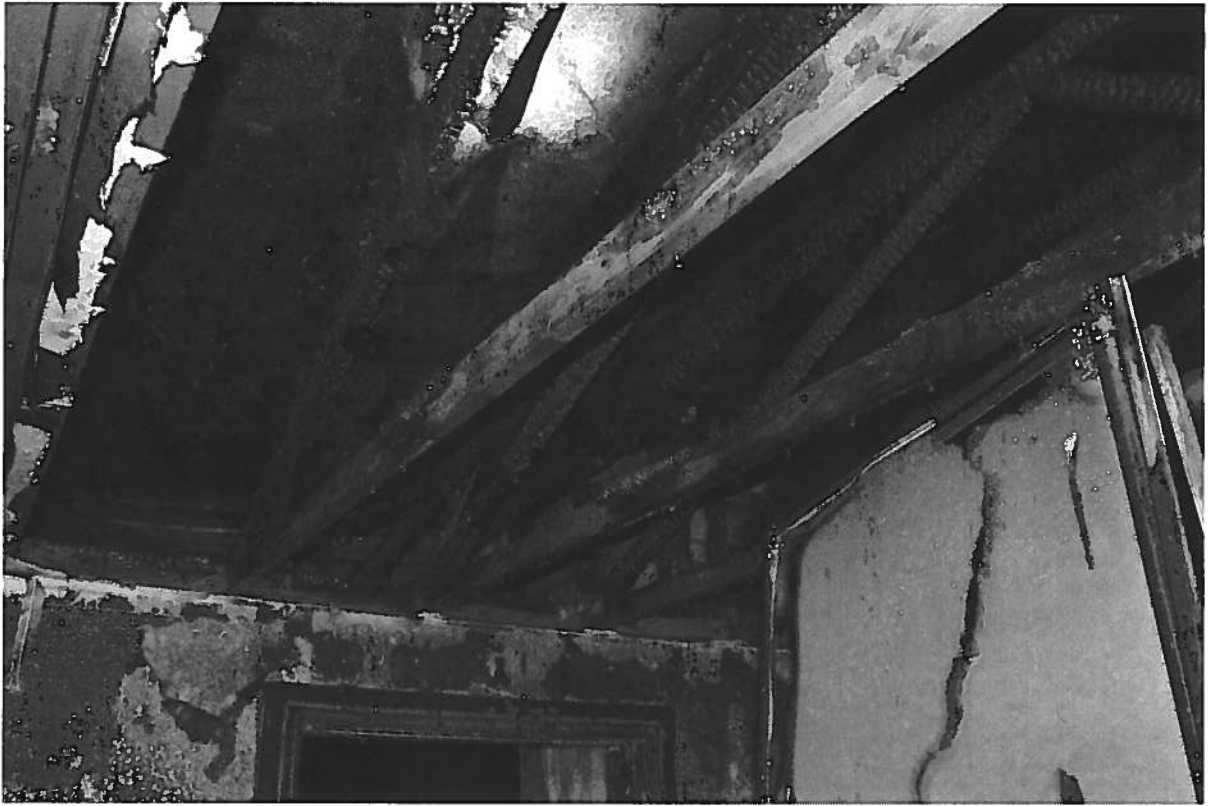
West Bedroom Attic
