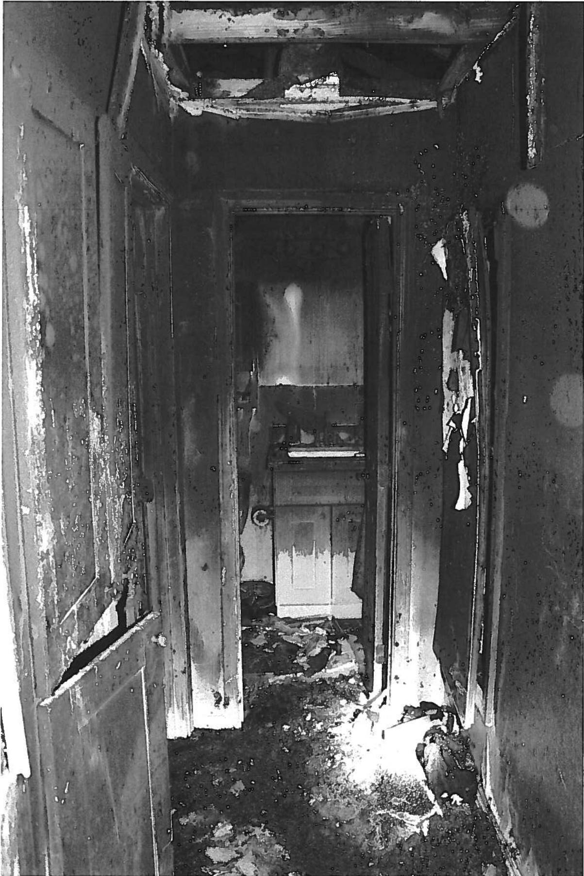
2 nd Floor Bathroom from Hallway
