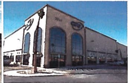
513,000-square-foot distribution center in NV
