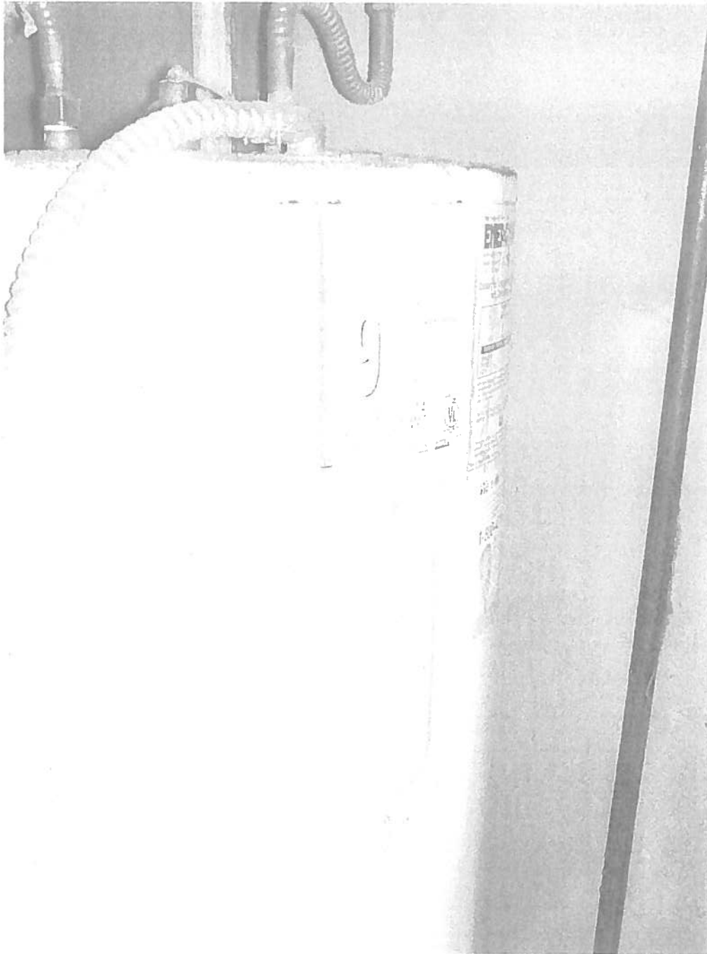
IP02 View of the water heater associated with the water supply to the restrooms.
