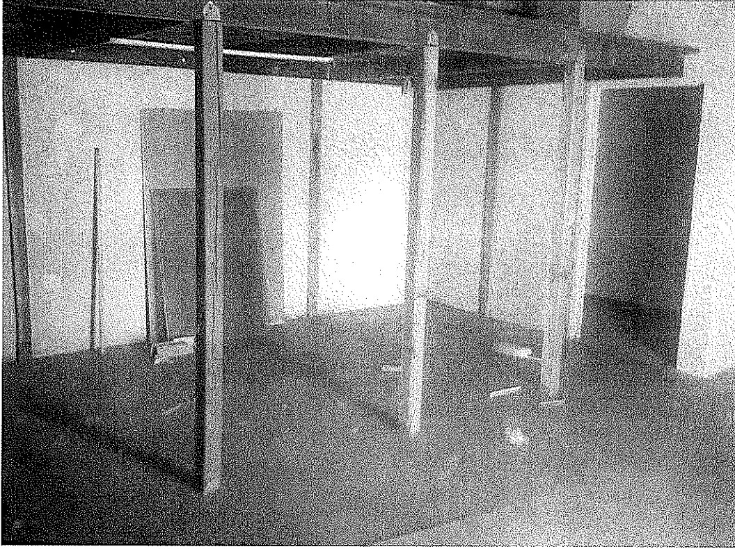
IP02 View of a rear storage room.
