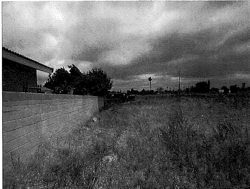
OP10 East facing view of northern boundary or property from the northwest corner.
