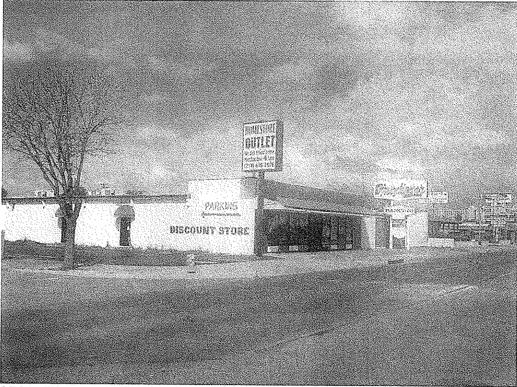
OP01 View of subject site at 12501 Harbor Boulevard, Garden Grove, CA.
