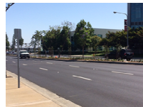
Euclid Street/median improvements
