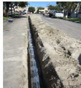
Water Improvements Buaro/Haster Strand Stone Gate Condos
