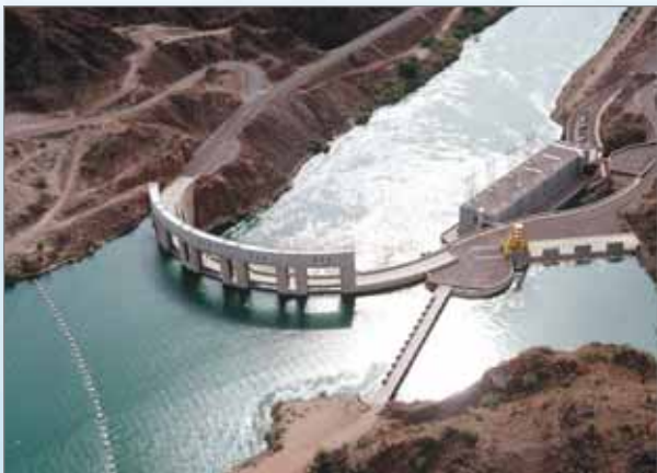
Imported water from the Colorado River travels over 240 miles to get to Orange County. Along the way, it is lifted over 1,600 feet by a series of five pumping plants. Shown here, near Parker Dam on the Colorado River, the Gene Pumping Station boosts the water over 300 feet. From there, it flows through a series of canals, pipelines, and tunnels across the Mojave Desert and beneath the San Jacinto Mountains on its way to fill the needs of the people of Southern California.
