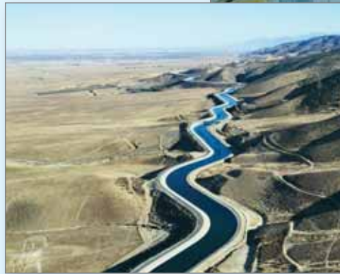
the State Water Project. Shown here, water is brought from Northern California via the State Water Project aqueduct system, then lifted over the Tehachapi Mountains at a rate of millions of gallons per minute on the way to southern California.
