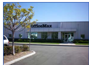
Office Max located in the Industrial Zone
