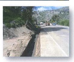
The Project consisted of the replacement and upgrading of water infrastructure within the Carbon Canyon Road and Olinda Avenue area, within the City of Brea, which included approximately 3,400 lineal feet of 6-inch DIP water line; approximately 300 lineal feet of 12-inch steel water line; various pump station upgrades, a retaining wall and surface restoration improvements.
