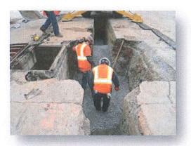
The Project consisted of the replacement of approximately 1,800 lineal feet of 8-inch DIP Water Line throughout Midbury Tract, in the City of Brea, including appurtenant pressure regulating infrastructure, gate valves and fire hydrants and associated pavement and concrete improvements.
