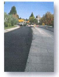
KOA provided complete construction management and inspection services for this \$7 million residential and arterial pavement rehabilitation project. Work included repair of concrete curb, gutter, sidewalk, cross gutters, and driveways; pavement repairs; edge grinding; asphalt rubber hot mix overlay; striping and markings; and traffic signal loop detectors.
